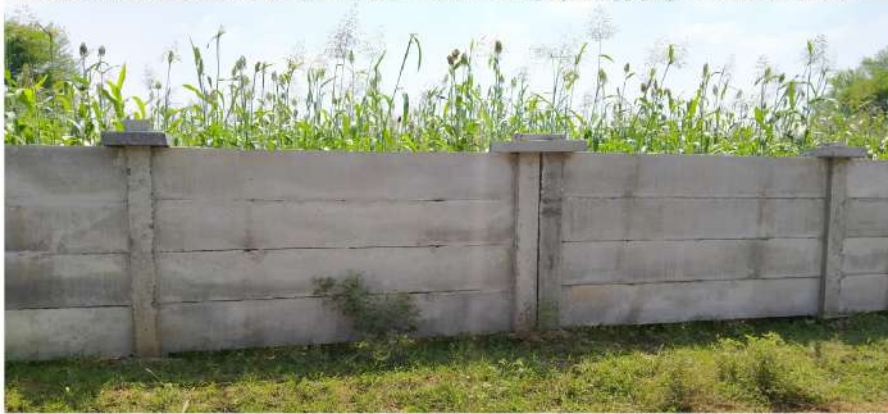
Boundary Wall @ L&T (DFCCIL Project) 70KM
